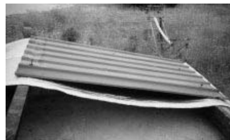
Figure 2 Experimental pitched roof with reflective insulation
