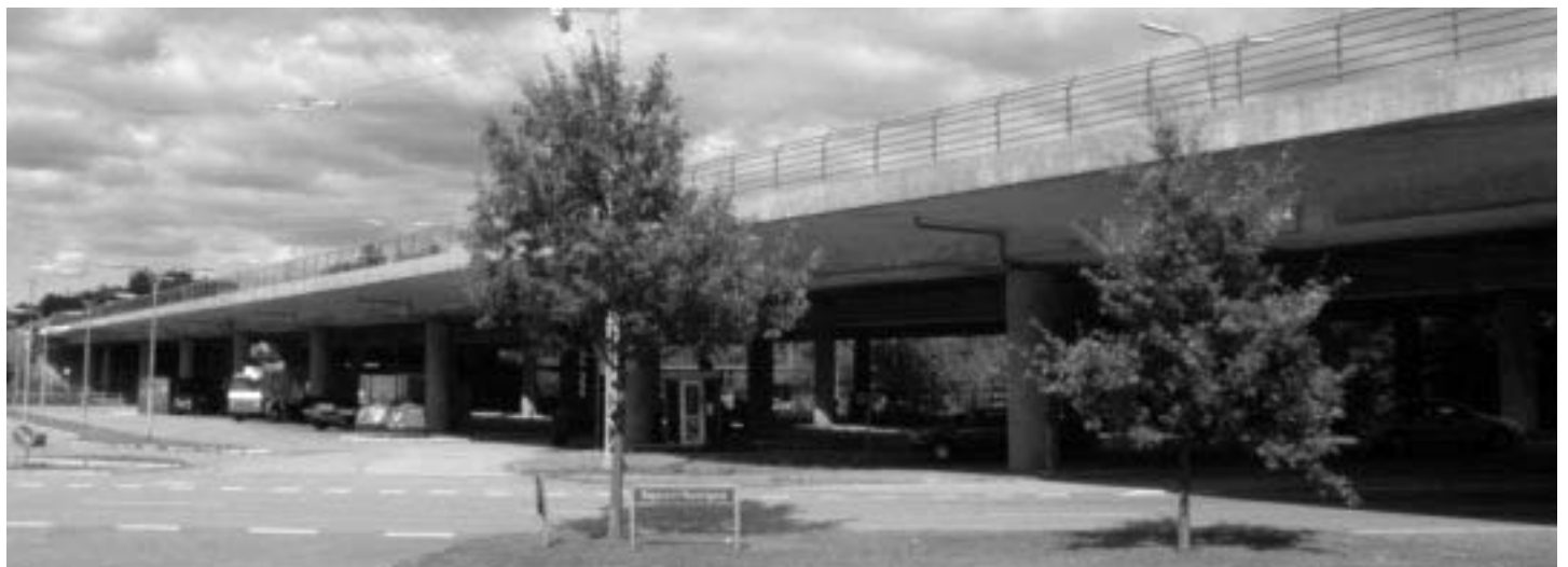
Monitored 'Skovdiget' bridge north-west of Copenhagen
