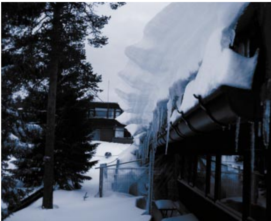
Winter in Oslo (photo: Thomas Thiis, Norwegian Building Research Institute)
