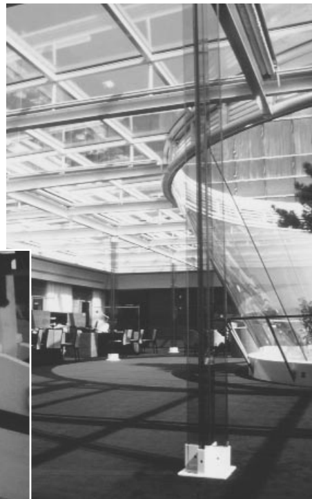
Administrative complex, Saint Germain en Laye: glass beams support a 700 square metre glass roof
