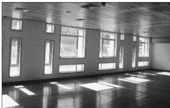
Interior view of the 'split window pattern'
