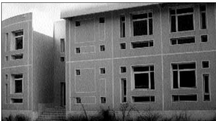
Pharmacy Faculty West Façade: 'split window pattern' for additional summer protection
